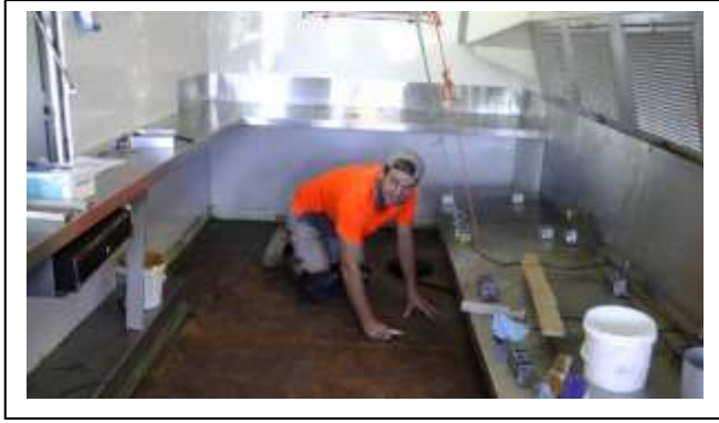
Our contractor preparing to lay the new floor
